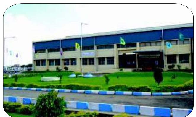
Engineering Products Plant Pashamailaram, Andhra Pradesh
