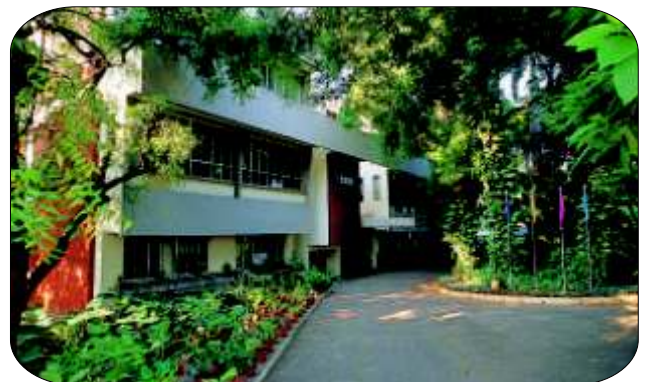
Belts and Oil seals Plant Madurai, Tamilnadu
