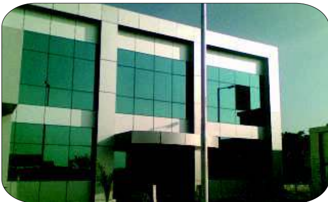
State-of-the-art R & D Centre, Sriperumbudur, Tamilnadu
