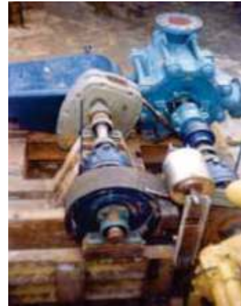
Hydro Testing Equipment
