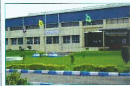
Engineering Product Plant, Pashamailaram - Telangana State
